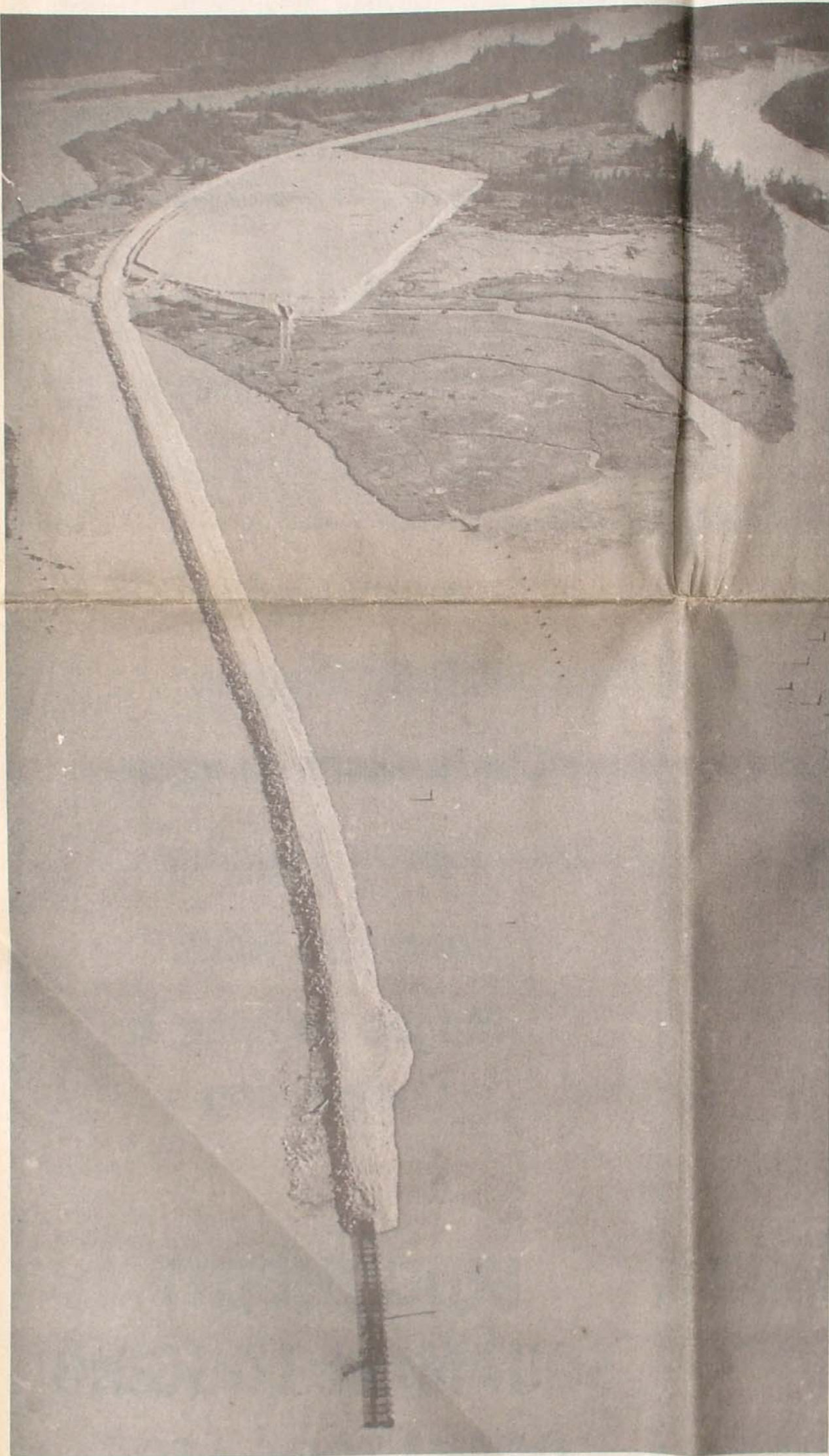
Training dyke at the mouth of the Squamish River
